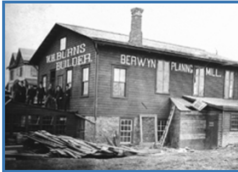
The W. H. Burns Planing Mill (ca1900-05, TEHS, 1996)
