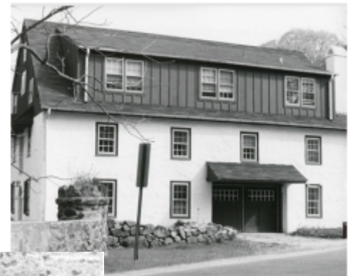
Mill Building (NPS)
